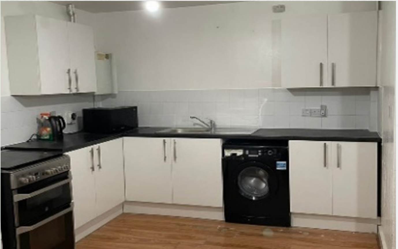
New Kitchen at Hale End Road This is one of 2 new kitchens we installed in 2023/24
